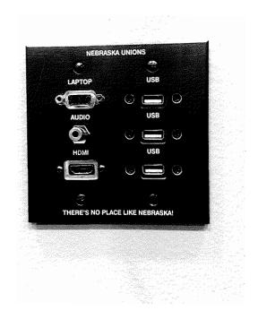
Below is the AV panel in the Gaughan Center. It is located right below the projection screen. When you arrive the Projector Off button will be red. Push the Projector on button and the projector will turn on and again please give it a few minutes to warm up and begin projecting. This is the setup in Ubuntu/Room 202 and Unity/Room 212.
